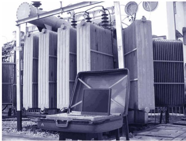
Fig. 6. On-site testing of a 33/11 kV, 6.3 MVA transformer using the developed setup.
